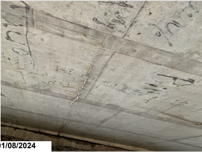
Typical soffit-under surface cracks.
