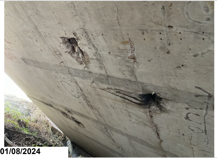
Span #1 soffit-under surface spalls with exposed rebar.
