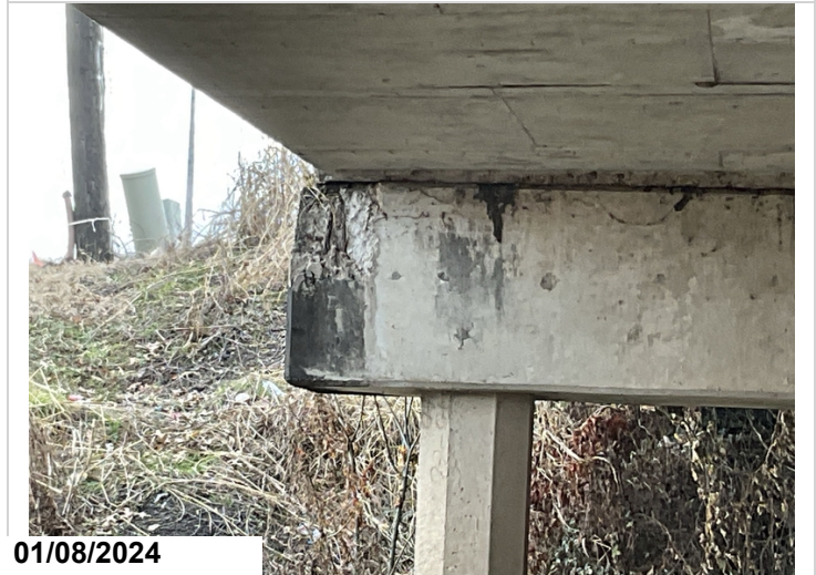
Bent #2 cap typical spall on ahead face
