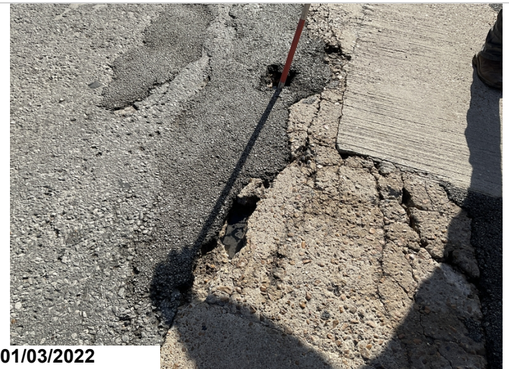
Span #3 left side between lanes has several areas spalled into the sona tube voids
