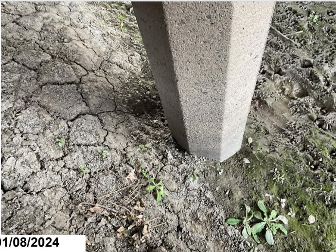
Typical abrasion on piles
