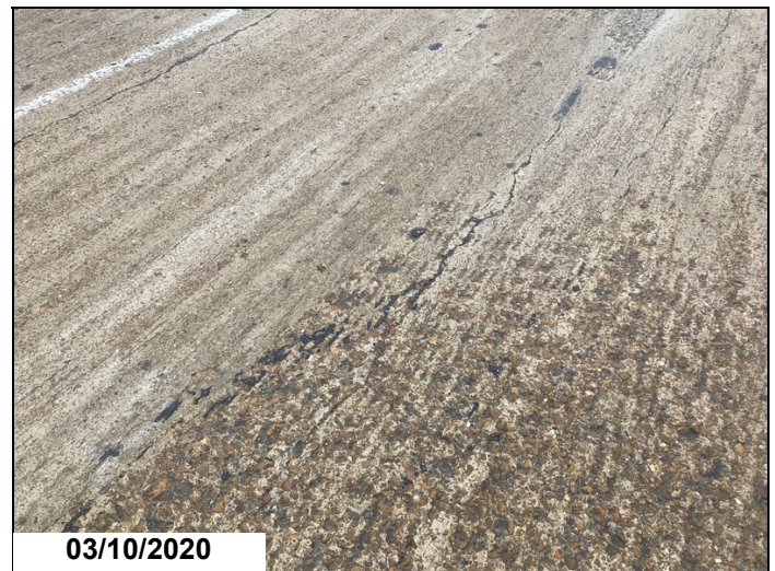
Typical longitudinal crack in deck.
