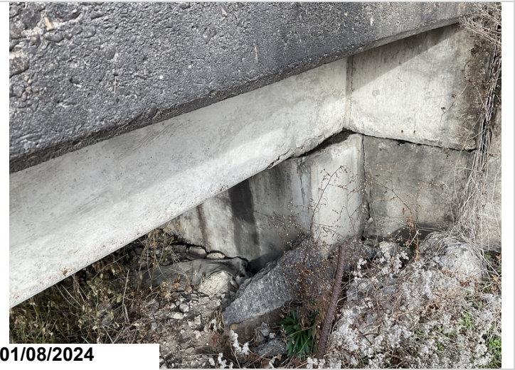
Slab right side at abutment #2 bottom edge has a 1' long crack delaminated area.
