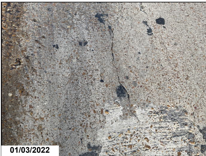
Typical longitudinal deck crack
