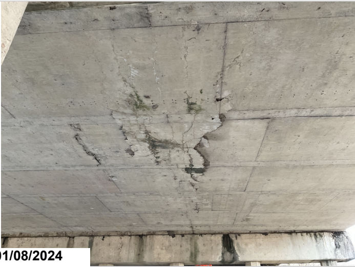
Span #2 soffit-under surface delaminated area.
