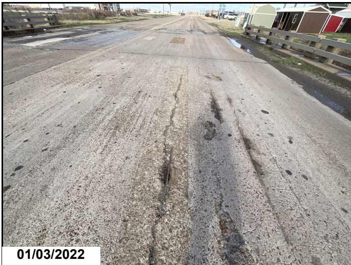
Span #2 exposed rebar in right lane
