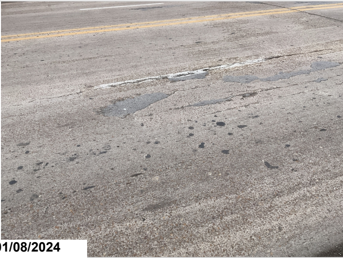
Typical deck cracks
