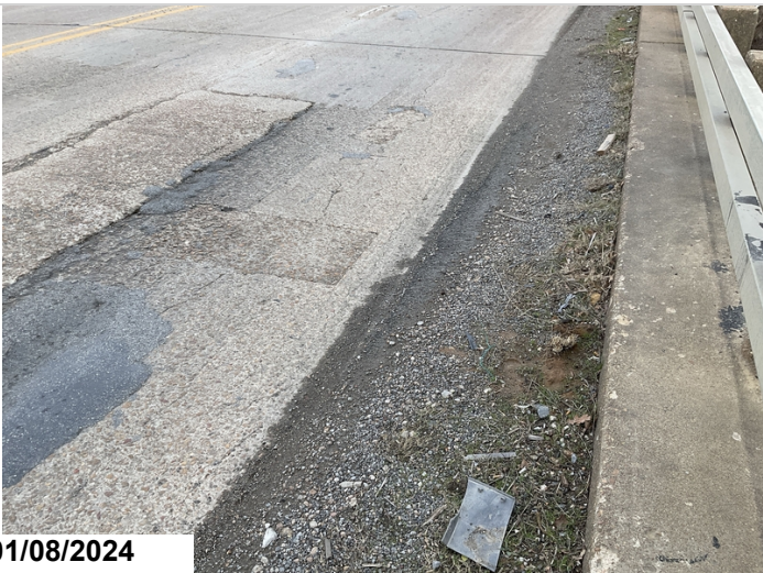
Typical debris in gutters
