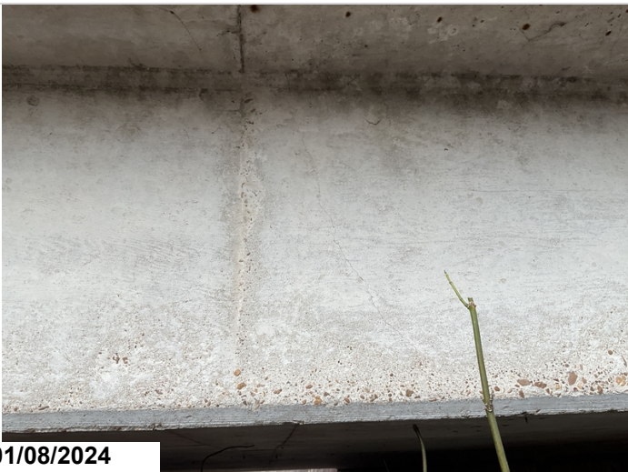
Typical cracks on sides of slab
